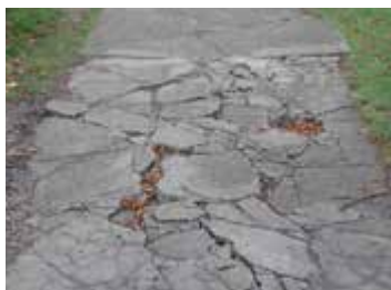
Example of a sidewalk needing replacement
